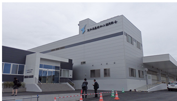
New office completed (left) and the refrigerated warehouse under construction (right)
