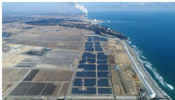
Second-phase construction; Haramachi Higashi solar power plant
