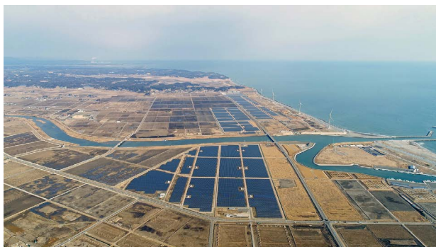
First-phase construction; Mano Migita Ebi solar power plant
