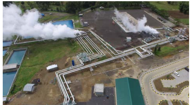
Steamfield Above-Ground System (SAGS) extending from the Ulubelu production well (Ulubelu power station [left] and Lahendong power station [right])
