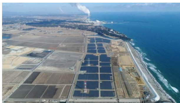
Second-phase construction; Haramachi Higashi solar power plant
