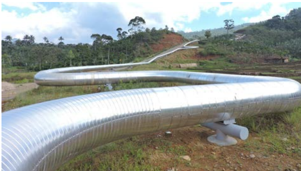
Steamfield Above-Ground System (SAGS) extending from the Ulubelu production well (Ulubelu power station [left] and Lahendong power station [right])
